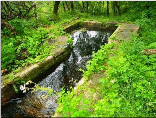
Photograph 2: Remains of original hydro-scheme intake
