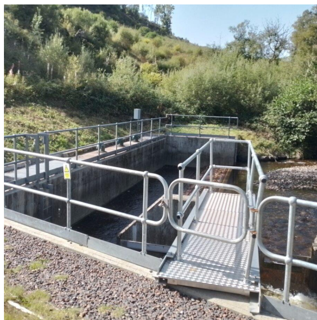
River Avich Hydro Scheme September 2023
